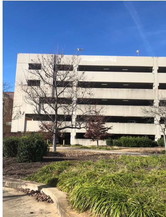
Parking Garage facing Martin Luther King Jr. Blvd
